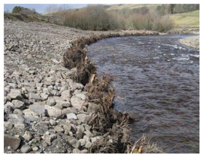
Engineered 'log jam' - soft engineering solution preventing erosion of the nationally important Tynebottom Mine spoil (River Tyne and Tynebottom Mine SSSI). © Natural England /Simon Stainer
